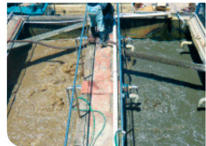
Operation in a aeration tank running condition
